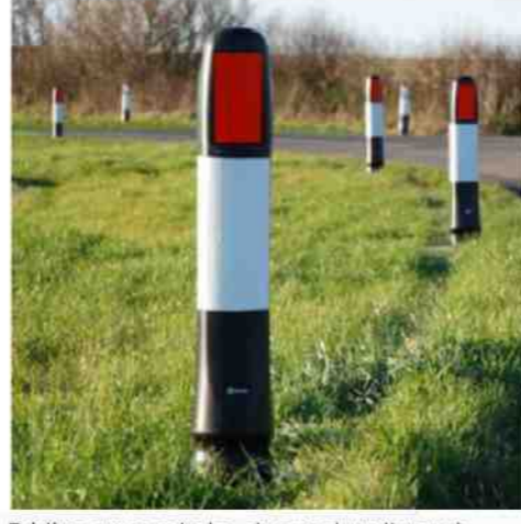
Existing access to be stopped up through installations of 600mm verge lined with Vergemaster Marker Posts and new access to be installed to county council standards
